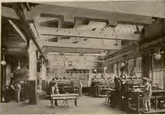
HOT-BLAST SYSTEM INSTALLED IN PRINTING ESTABLISHMENT
